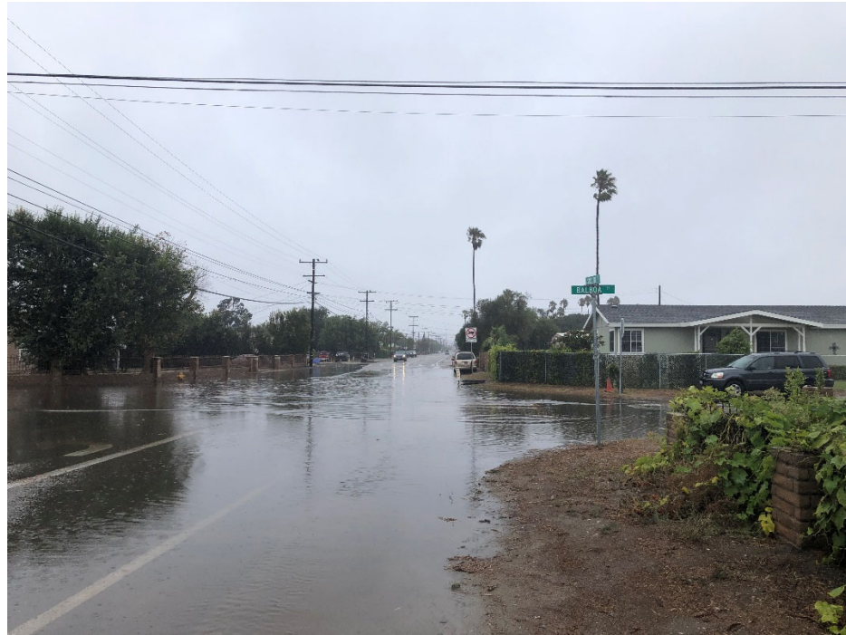
Storm event on 10/25/2021 with 0.75" water in the El Rio community
