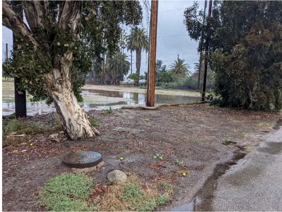
Storm event and flooding on 12/23/2021 in the Saticoy community
